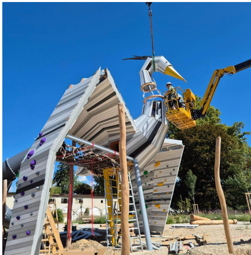
Regeneration of 2.35 hectares of green space Heron-themed playground structure.
